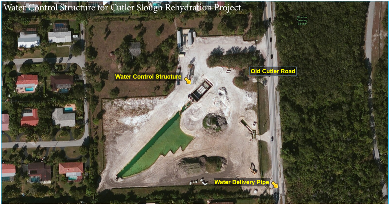
Overview of Cutler Slough Rehydration Project
